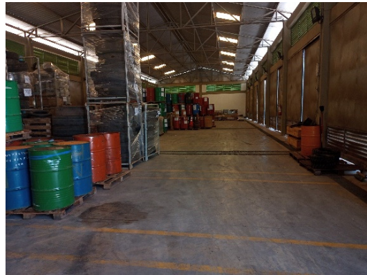
Figure 2: Hazardous waste storage facility (Class I) – internal view.
