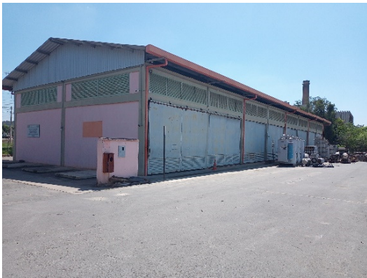
Figure 1: Hazardous waste storage facility (Class I) - external view.
