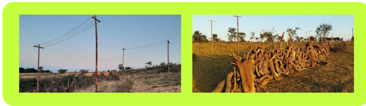
Wooden perches connected by cables
