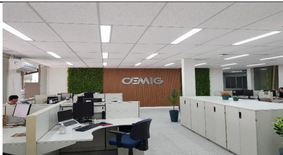
Figure 1: Retrofit of facilities with LED lighting.
