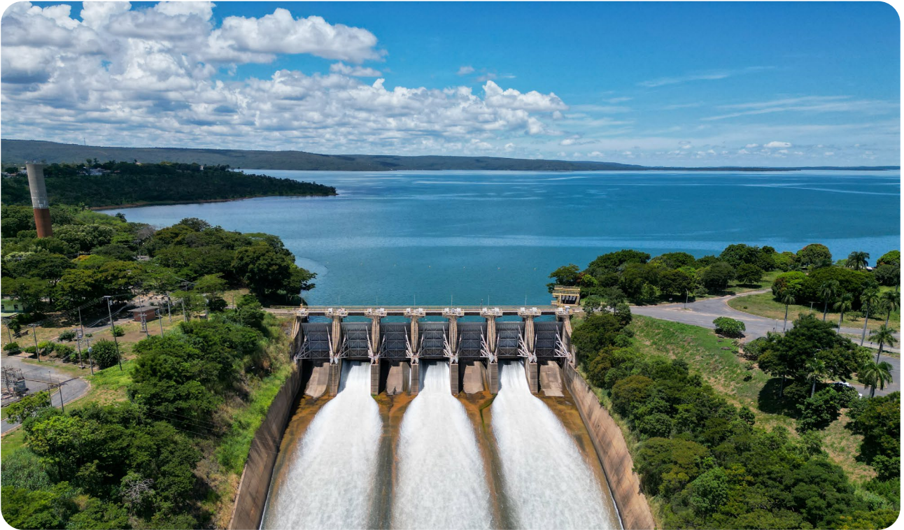
Três Marias Hydroelectric Power Plant
