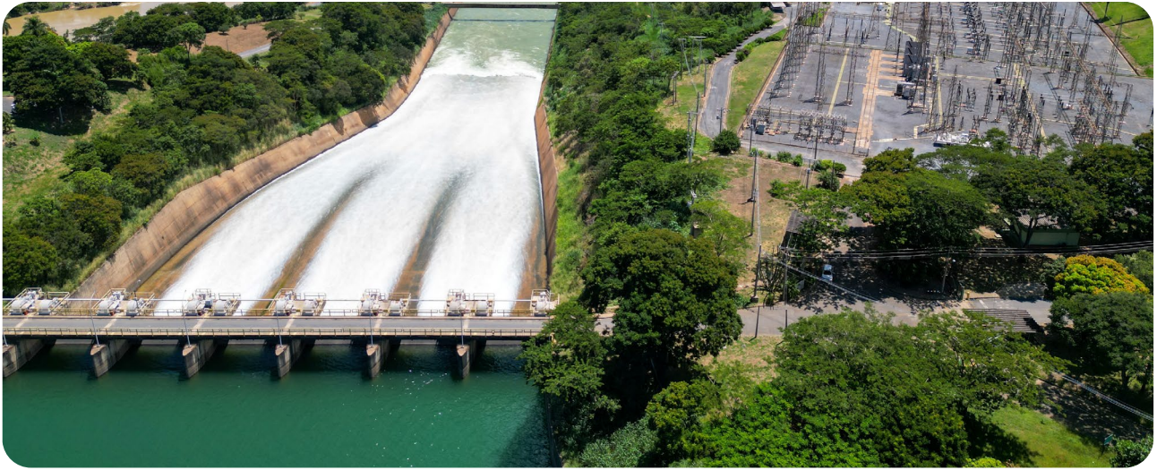
Três Marias Hydroelectric Power Plant
